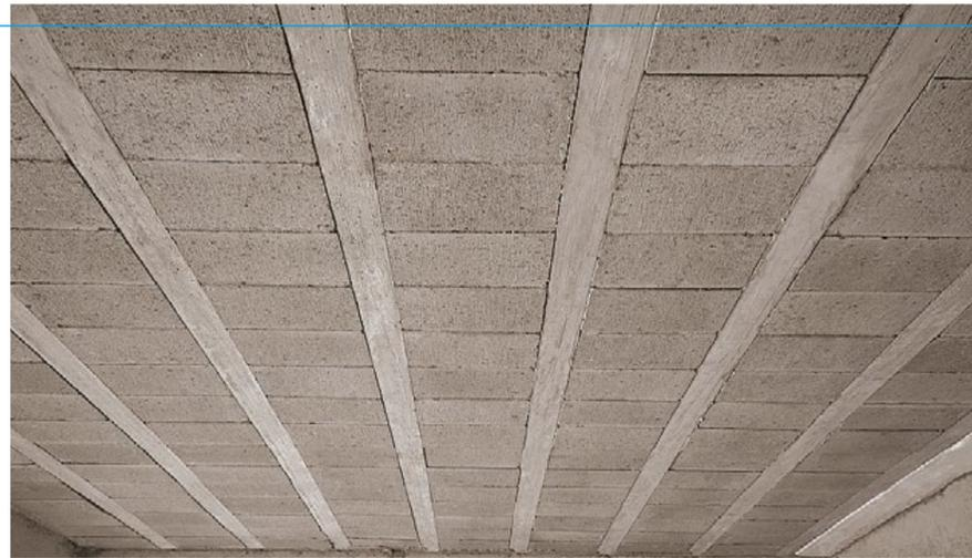
DETALLE MIX (BANDEJA DE CONCRETO CON BLOQUE RECTO POLIESTIRENO)
